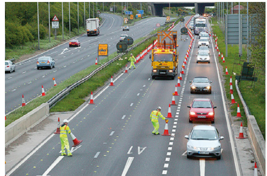
Figure 16 Intelligent road cones on a motorway
