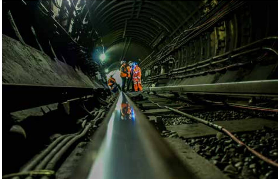
Researchers from CSIC and engineers from London Underground using a 3D laser scanner to measure deformations in the London Underground Northern Line station at Euston. The photograph was taken by DIAL's Dr Phil Catton and it won third prize in the Engineering Department annual - and fiercely contested - photography competition.
