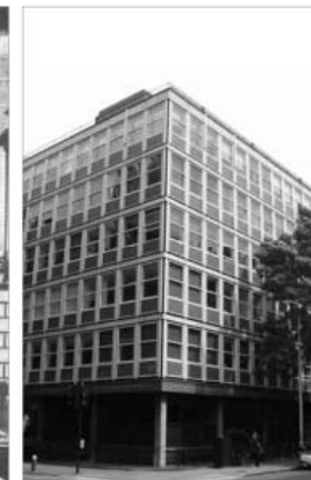
(b) 1950s, Deep foundations
