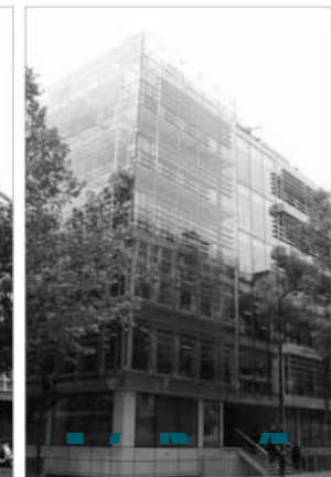
(c) 2002, Reused foundations (refurbishment)
